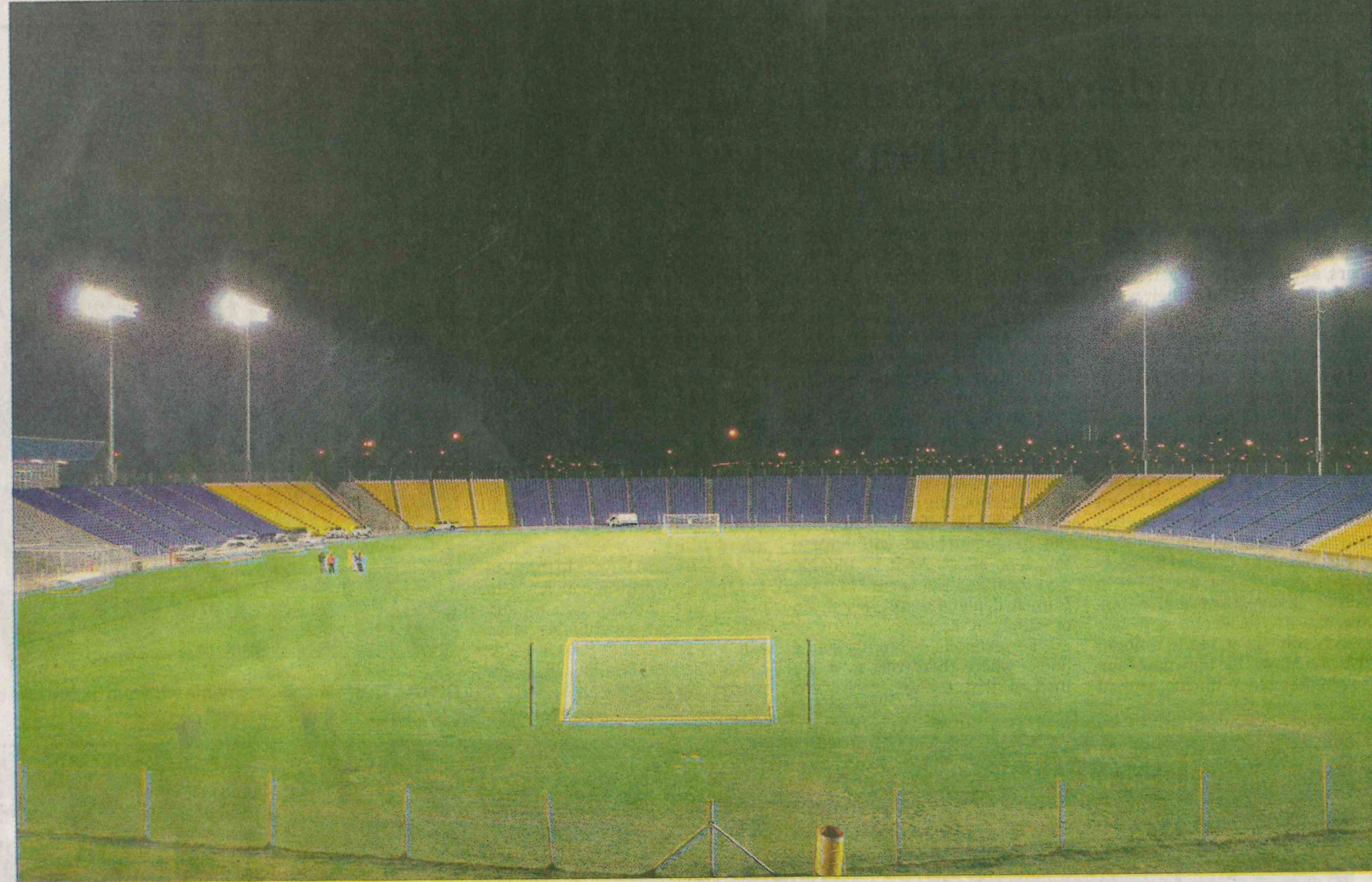
LIT UP: With its new lighting system, Kaizer Sebothelo Stadium in Botshabelo is now equipped for HD television broadcasting.
